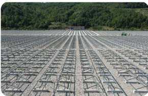
Construction of photovoltaic structures 2023
