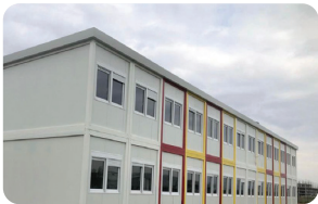
School construction in Skopje 2021
