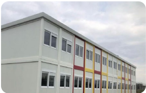
School construction in Skopje 2021
