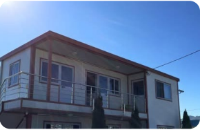
2008 Construction of new facilities
