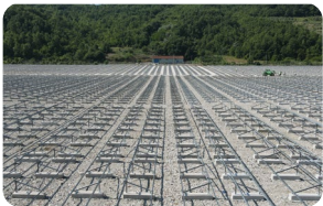
Construction of photovoltaic structures 2023
